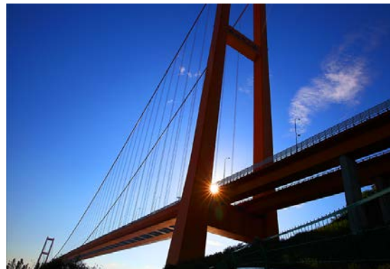
Basac River Bridge Completed
