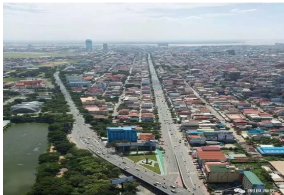
The 51 National Road Construction Started
